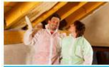
Attic Air Sealing ▶
